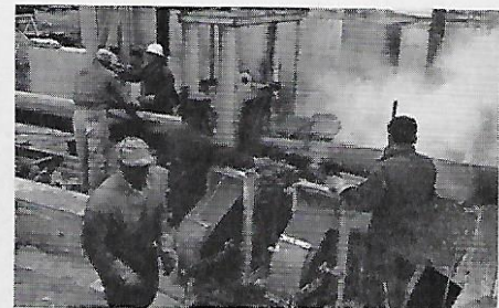
Coated with layers of asphalt and felt
