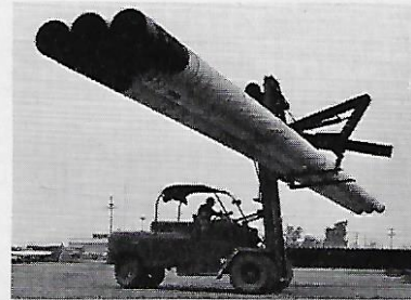
And dispatched to the Junction-Oleum job.
